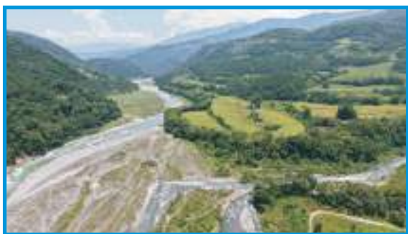
Siang river at Yingkiong
