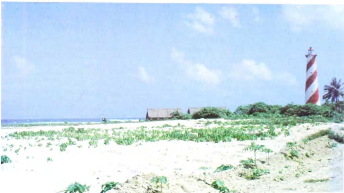
Fig. 11 : A light house at Pygmalion point, the southernmost point of Indian territory
