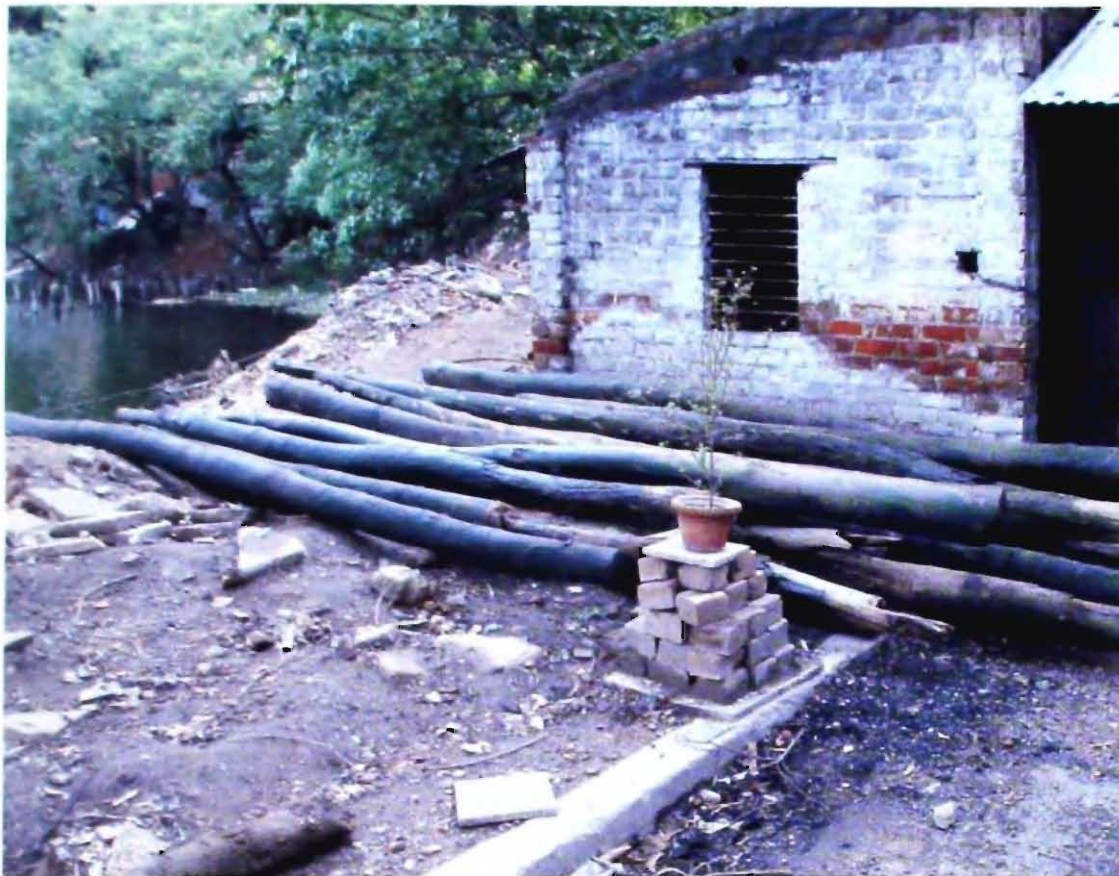
Fig. 6 : Showing demolition of residential quarter beside Indian Museum Tank
