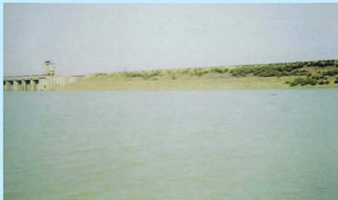
Figure 3 : A panoramic view of Tenughat Dam
