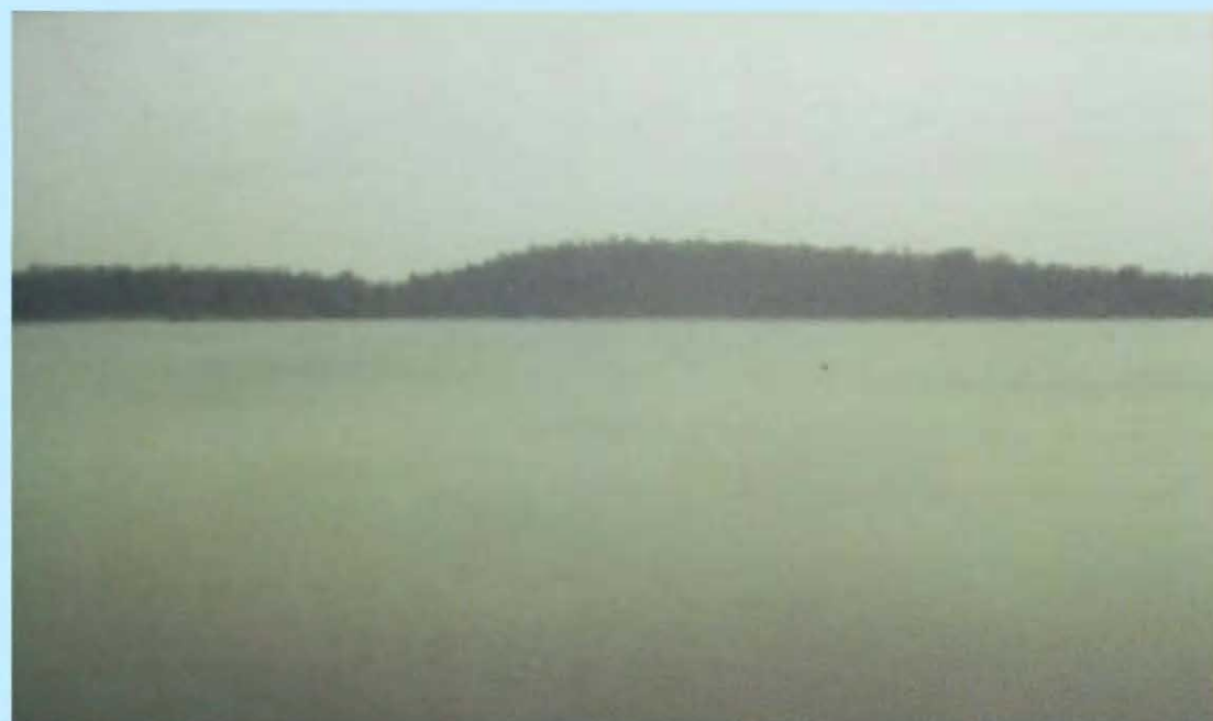
Figure 1 : A panoramic view of Tilaiya Dam
