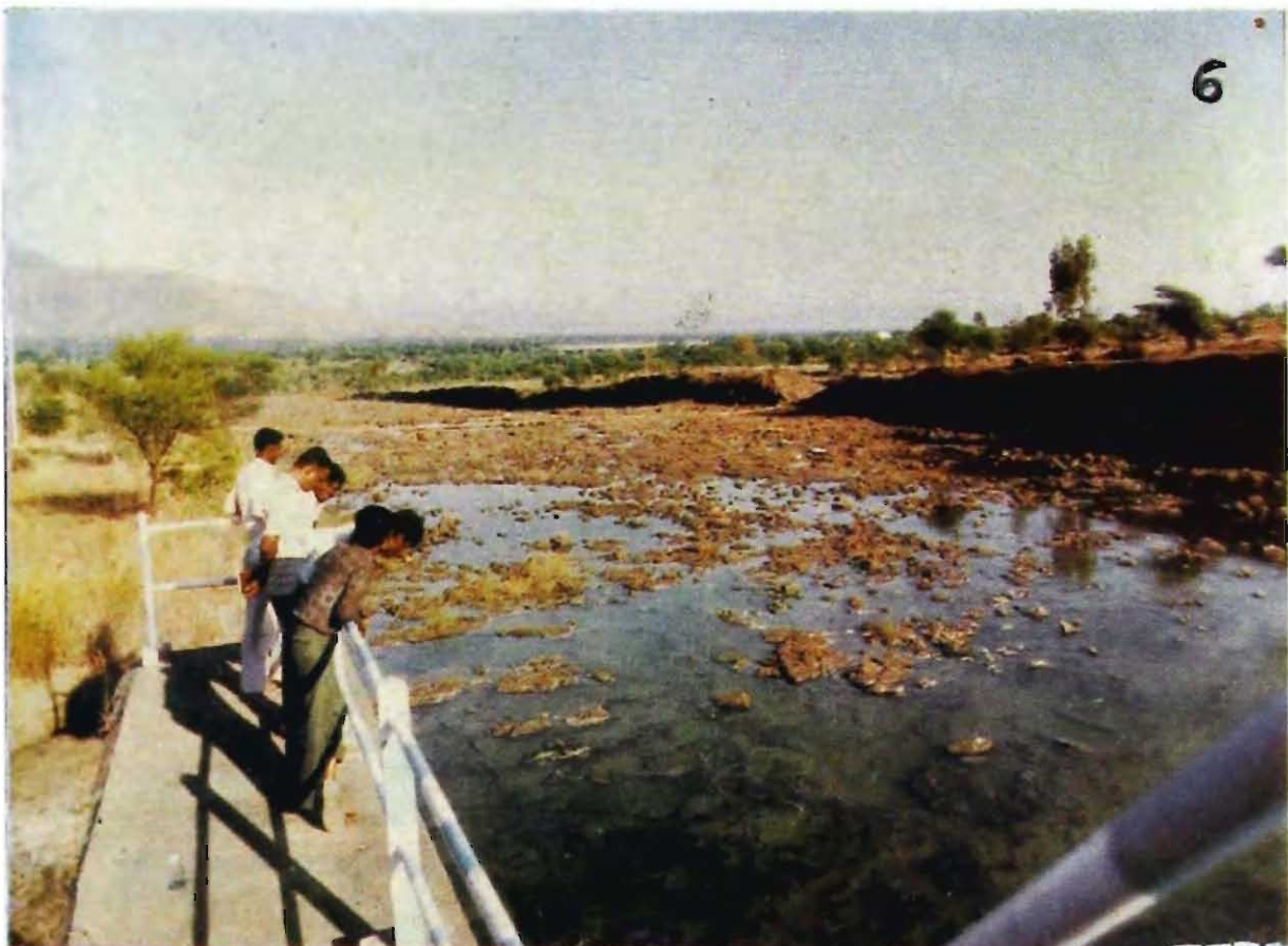
6. The original course of R. Krishna dammed and diverted at Dhom, 2.1.1988.
