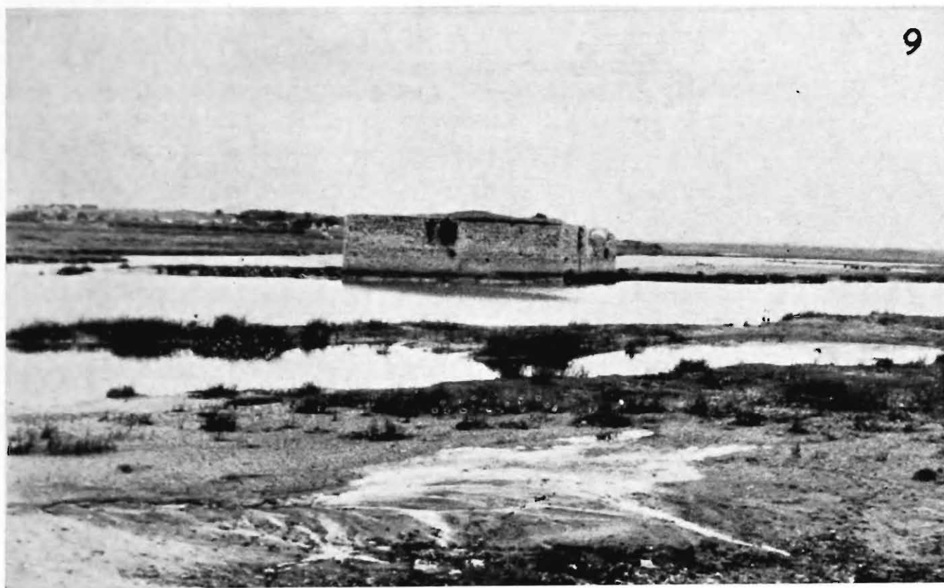
9. Upstream view of R. Tungabhadra, Nawab's Bungalow near Kurnool Town. 14.12.1987
