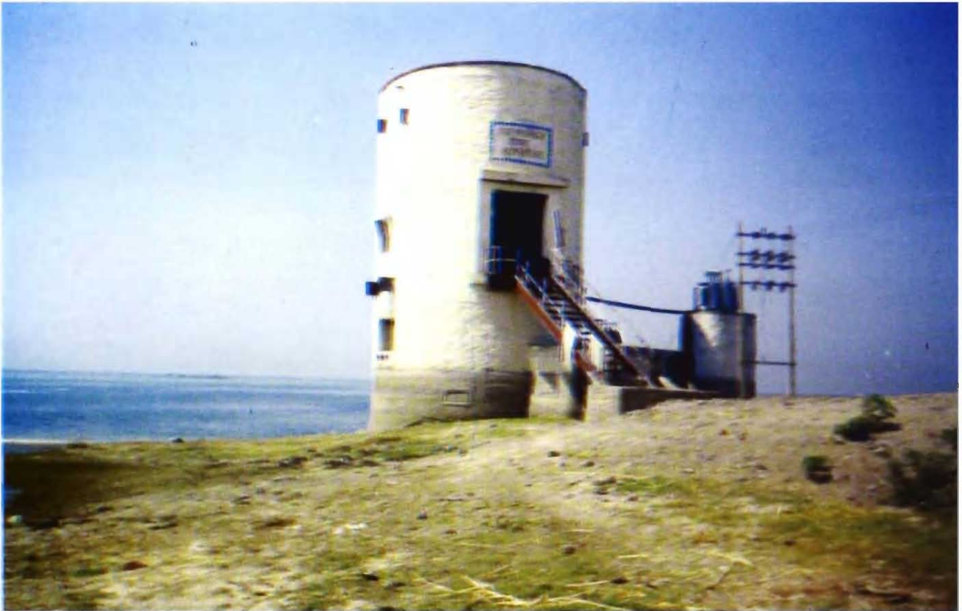
Pumping station on the bank of wetland
