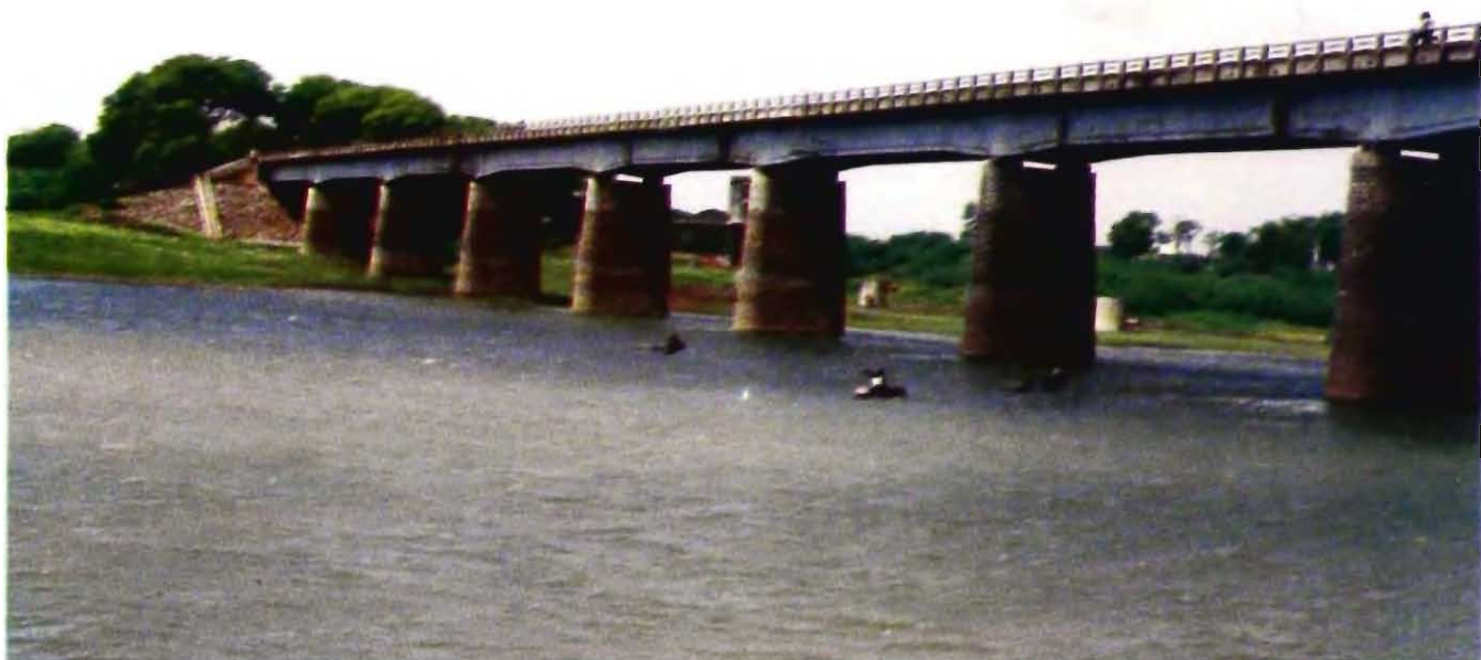
A bridge on Godavari river near Jalkwadi Project
