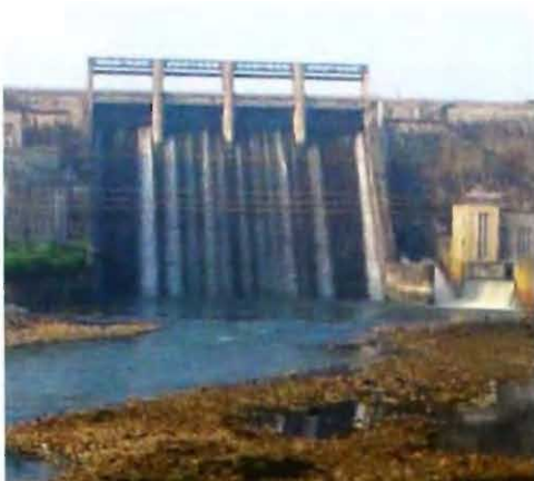
Bhadra Dam at Lakkavalli
