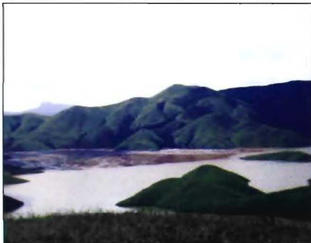
Fig. 3. Lakhya Dam reservoir filled with silt.
